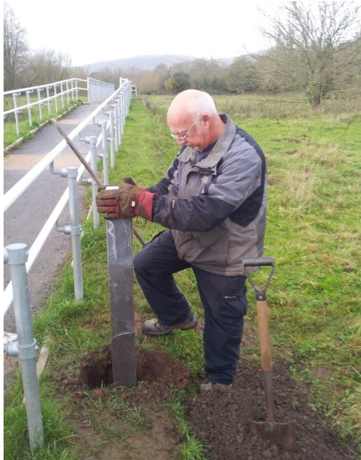
Field Warden installing a counter to monitor usage and inform grants.
